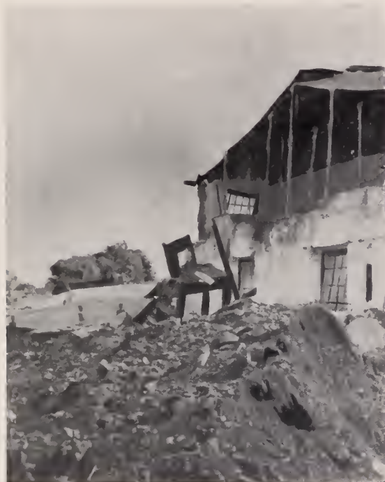
FIG. 1. EASTERN END OF FACTORY, DOLOI.
